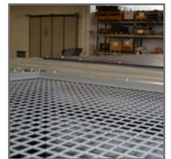
Air outlet louvres with metal mesh to protect the expulsion from leaves/dirt
