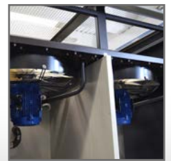
70 EDR* model VSD driven fan remote radiator properly sized for the temperature
