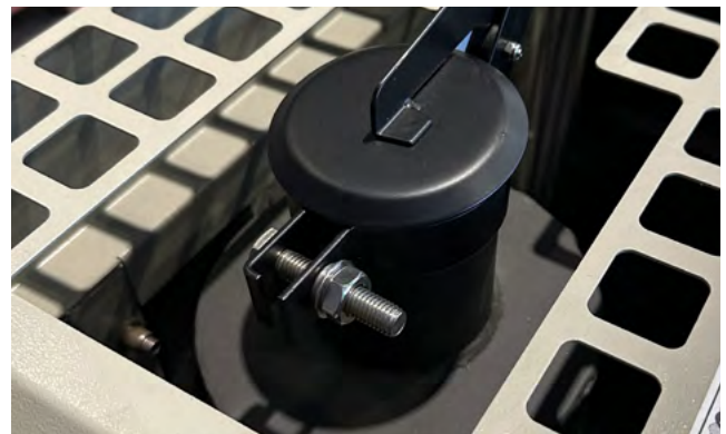
Residential muffler -35 dBA, equipped with exhaust terminal with self-closing rain cover
